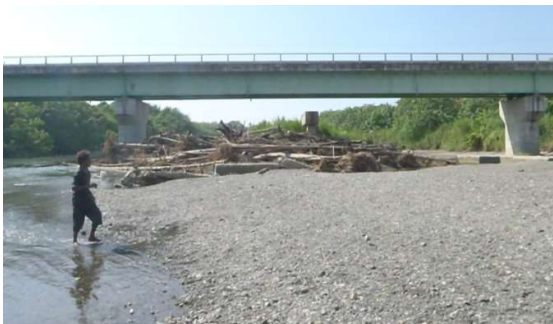
8E. Ngalimbiu bridge, viewed from upstream
