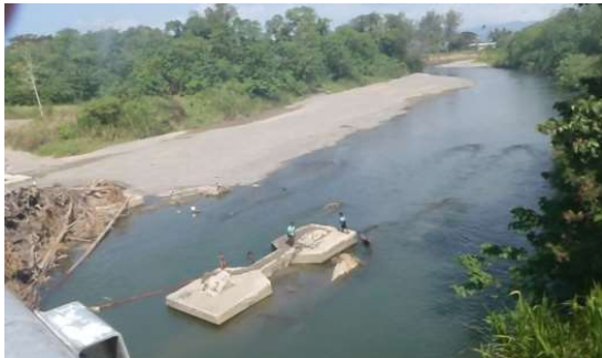
8C. Sand deposit on right bank – old pile
