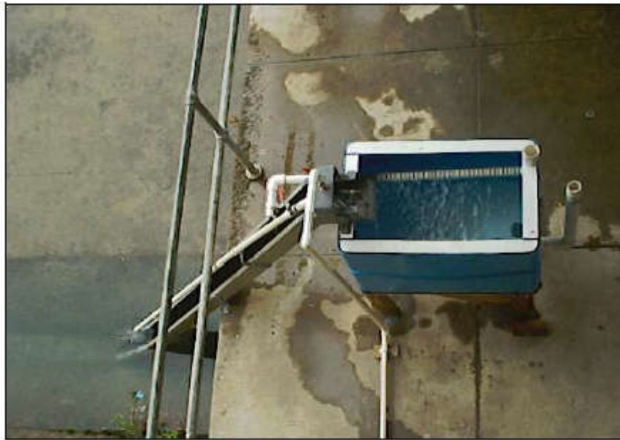
Figure 11-3 Photo of ramp and trap at dam
