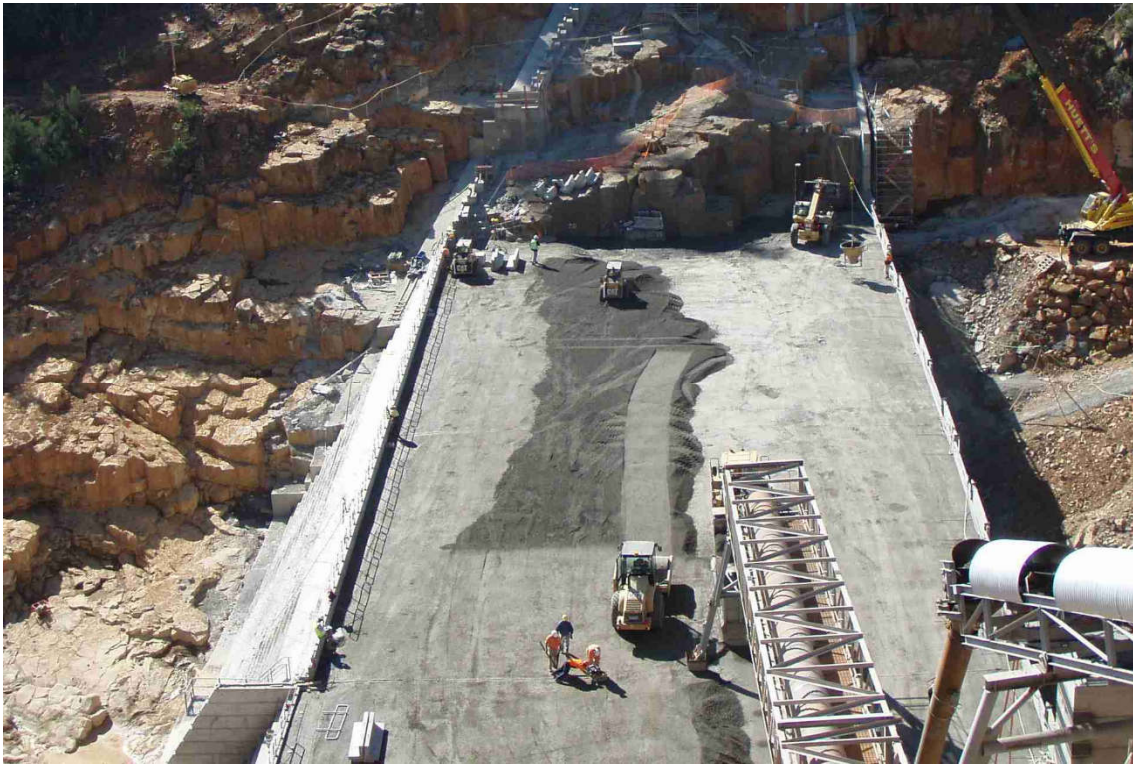
Figure 2-4 Typical RCC dam construction with concrete conveyor
