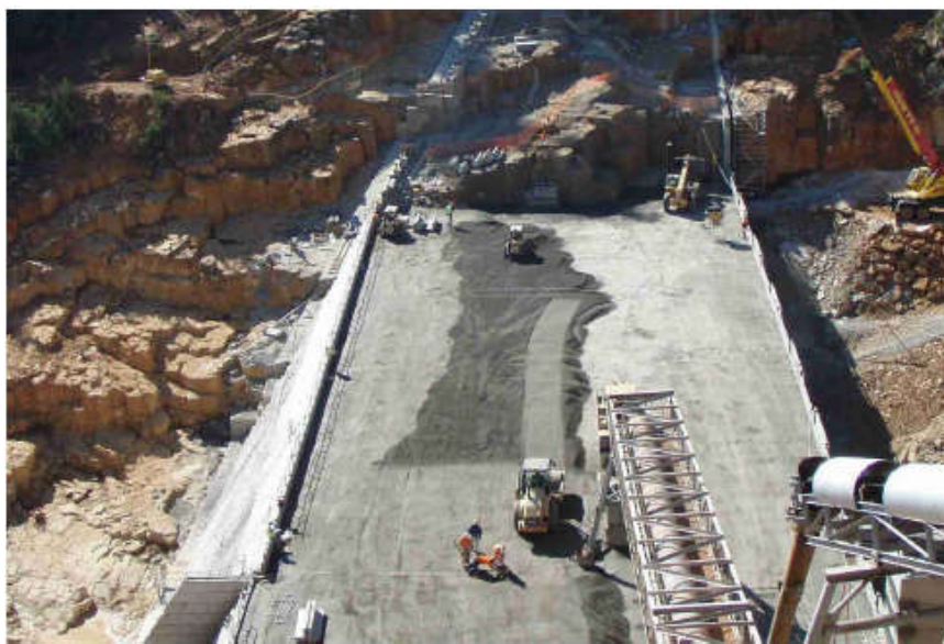
Figure E-0-5 – Example of RCC Dam Construction
