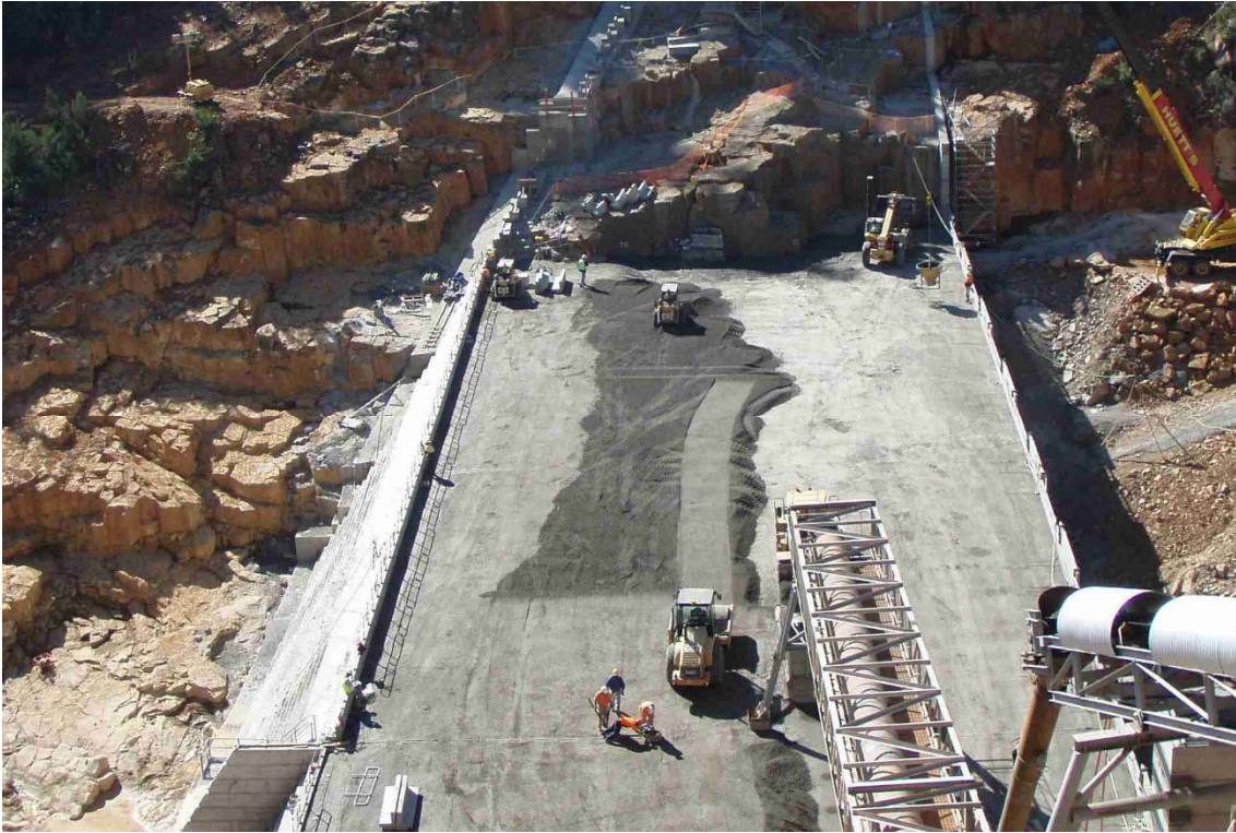
Figure 2-4 Typical RCC dam construction with concrete conveyor
