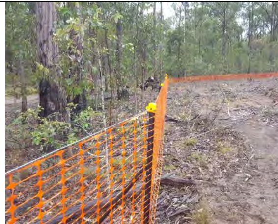
Figure 3-4: Vegetation protection fencing (Advanced Group 2024)
