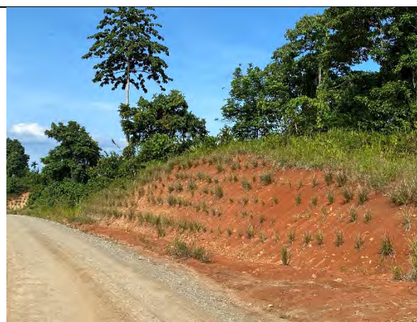
Figure 4-2: Vertiver grass planted along Lot 1
