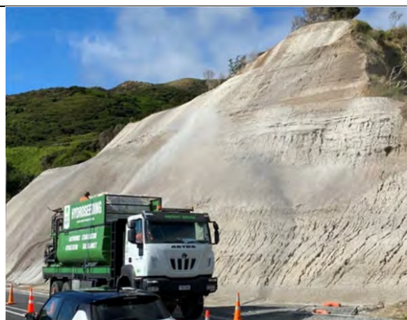
Figure 4-4: Hydroseeding can be used on steep terrain (Instant Green 2024)
