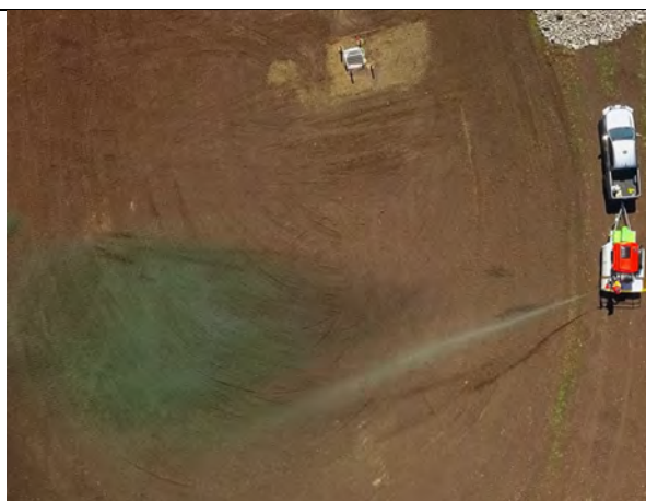
Figure 4-5: Equipment can be mounted on a ute, truck or trailer (Vortec 2024)
